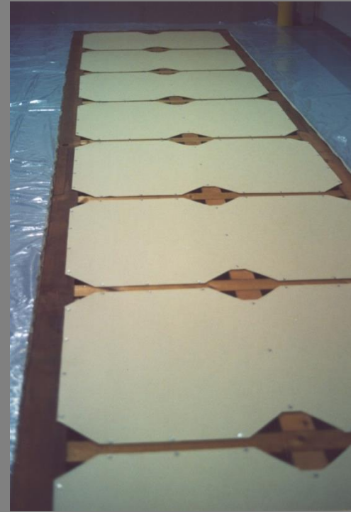
Vacuuming and removing debris and backing boards.
